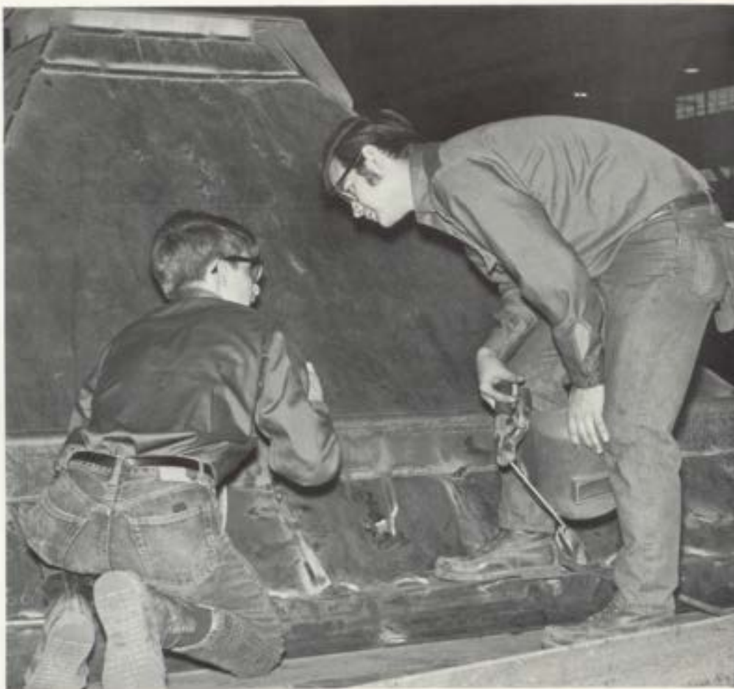
At Rex Chainbelt, Robert Hillenburg, an ICT student, and his supervisor, discuss welding a gravel bin that empties into a cement mixer.
