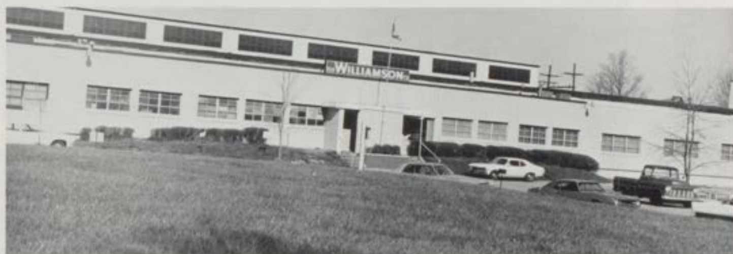
Serving since 1947, Williamson Heating and Cooling is one of Madison's oldest hilltop manufacturing plants, 1200 Clifty Drive.
