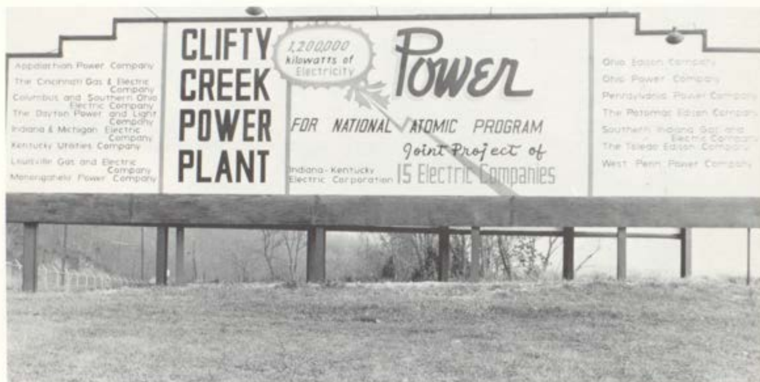
Madison Clifty Creek Power Plant this year undertook an extensive renovation program to increase power output.
