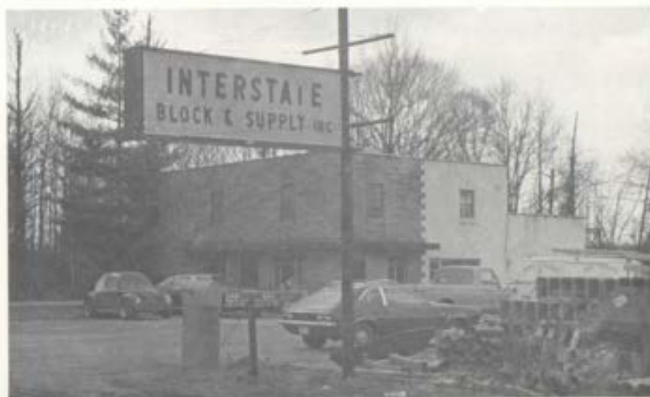
Blocks manufactured by Interstate Block and Supply Co. 3148 Clifty Drive comprise the foundations of most Madison homes.
