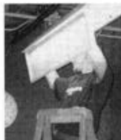
Danny Tullis changes out a bulb in the shop area.
